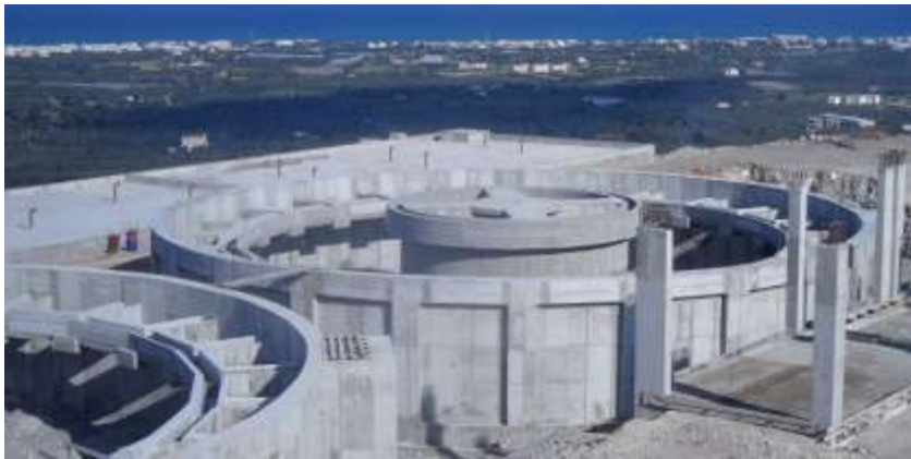
Construction of Settlement Tanks
